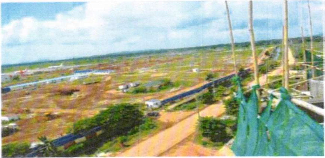
NITB Guwahati Airport Site:- 3 m Barricade Wall.
