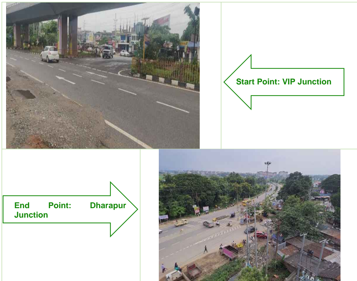
Photo 1-1 : Start and End Point for Airport Connect
