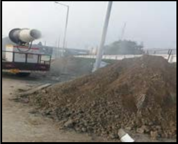
Water sprinkling on Soil before handling
