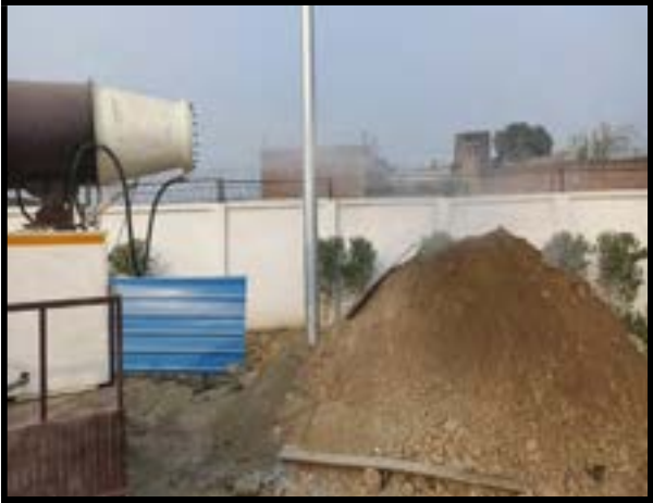
Water sprinkling on Soil before handling
