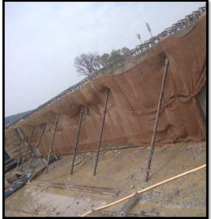
Use of hessian cloth to save water during concrete slab curing
